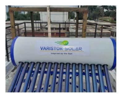
system features a robust Glass-Lined Coated (GLC) tank. This specialized tank not only contributes to overall efficiency but also extends the system's lifespan by preventing corrosion. The marriage of ETC technology and the GLC tank establishes the "200 LPD ETC GLC Varistor Solar™ Water Heater" as a premier choice, offering a harmonious blend of performance and longevity in water heating solutions.
